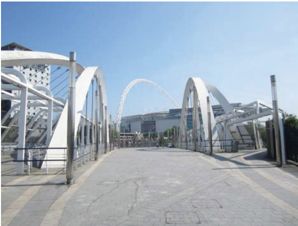
Picture 4.32 View of the Stadium from the White Horse Bridge
