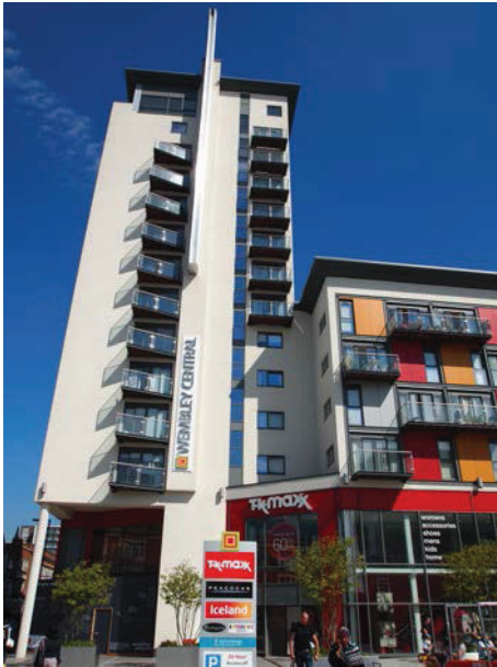
Picture 4.38 Wembley Central Square Development
