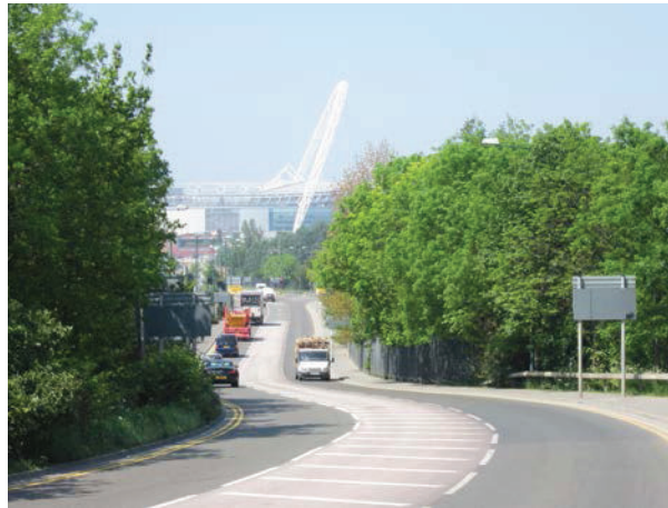
Picture 4.33 View of Wembley Stadium from the east
