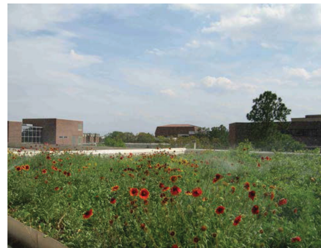
Picture 11.5 Example of a green roof
