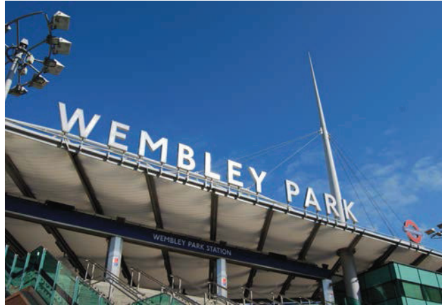
Picture 4.30 Wembley Park Station
